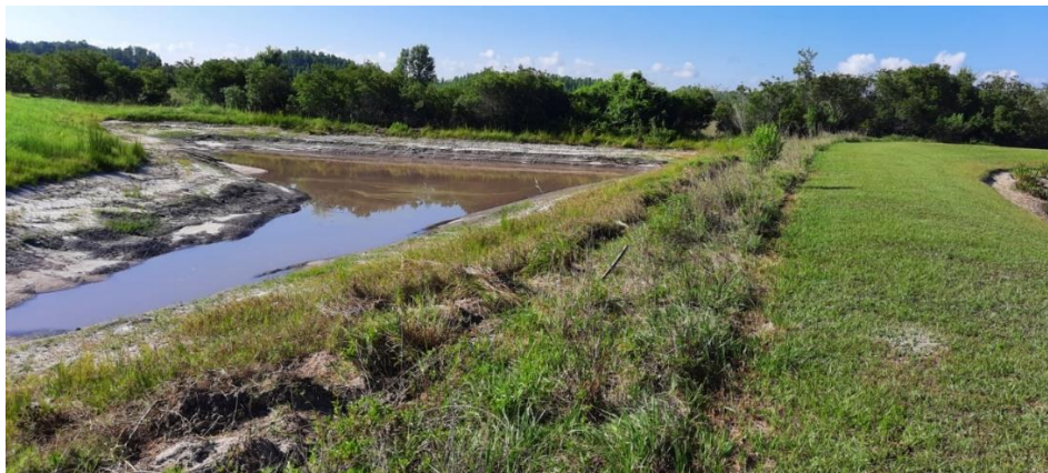
Looking south, Woodcreek CDD pond on left; MPIV CCD/Windsor pond on right – Need to verify CDD Boundary.
